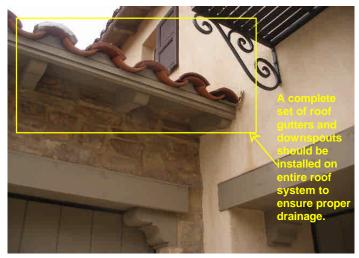
The roof needs to be cleaned to ensure proper drainage to prevent roof leaks. There may be bird droppings or other trapped leaves on rooftop that should be cleared.
